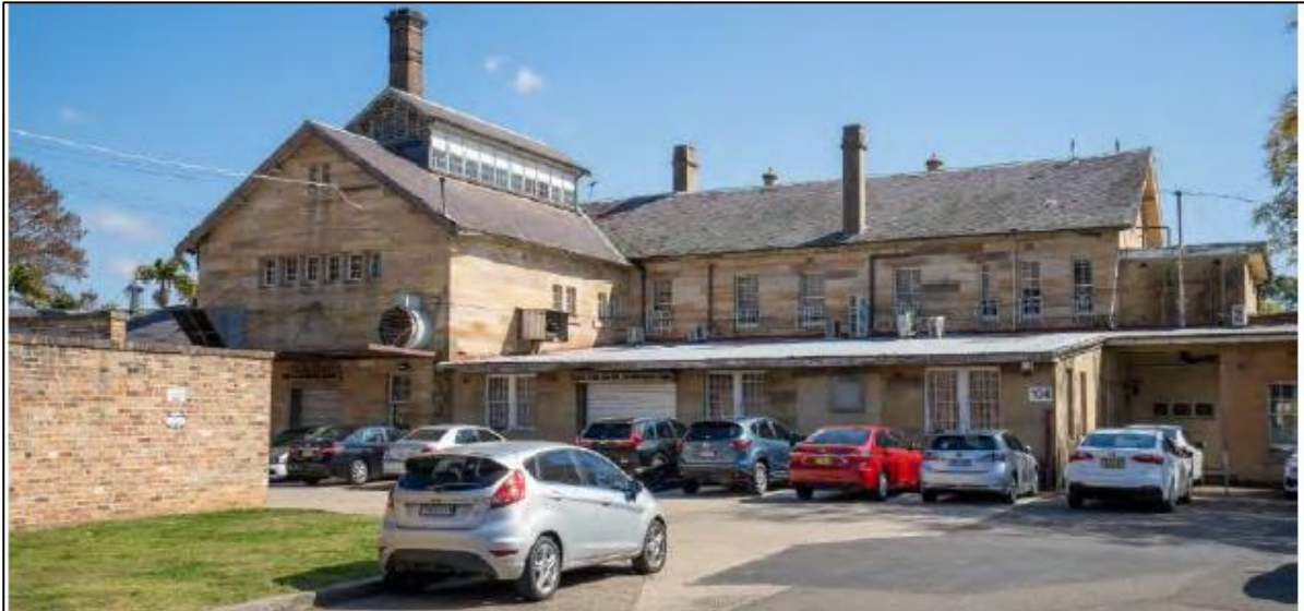
Figure 6: South elevation of building C104 (main Kitchen Block) (Source: TDK Architects)
