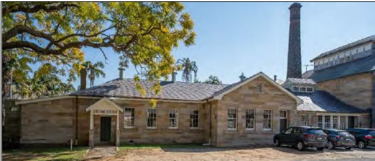
Figure 7: Part south elevation building C104A (Boiler House/Bathroom/Dining Room/Servery) (Source: TDK Architects)
